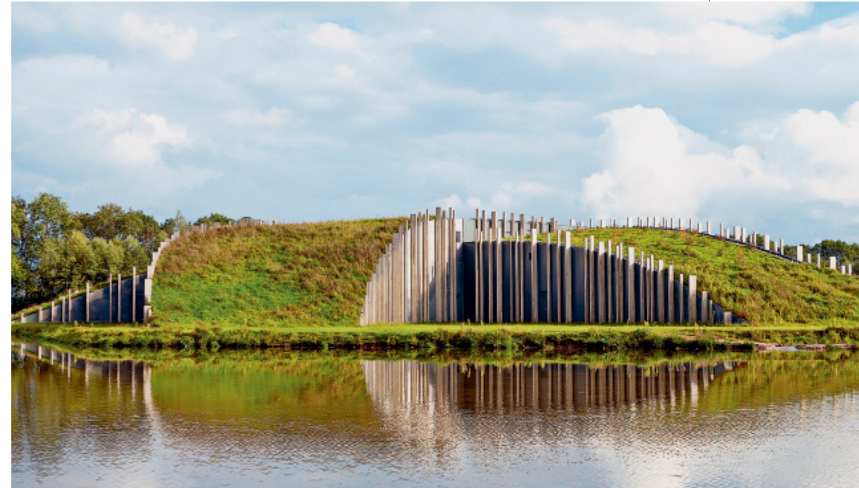
Production plant Vechterweerd near Dalfsen applies bank filtration. This plant provides drinking water to ten percent of the residents of the province of Overijssel.
