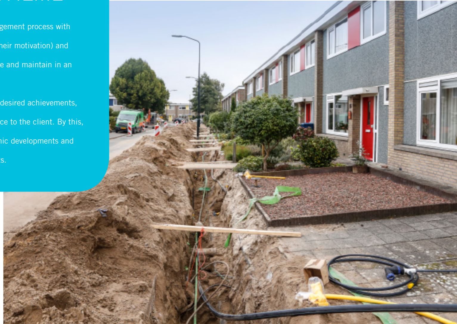
Vitens and Liander are replacing water and gas pipelines together
