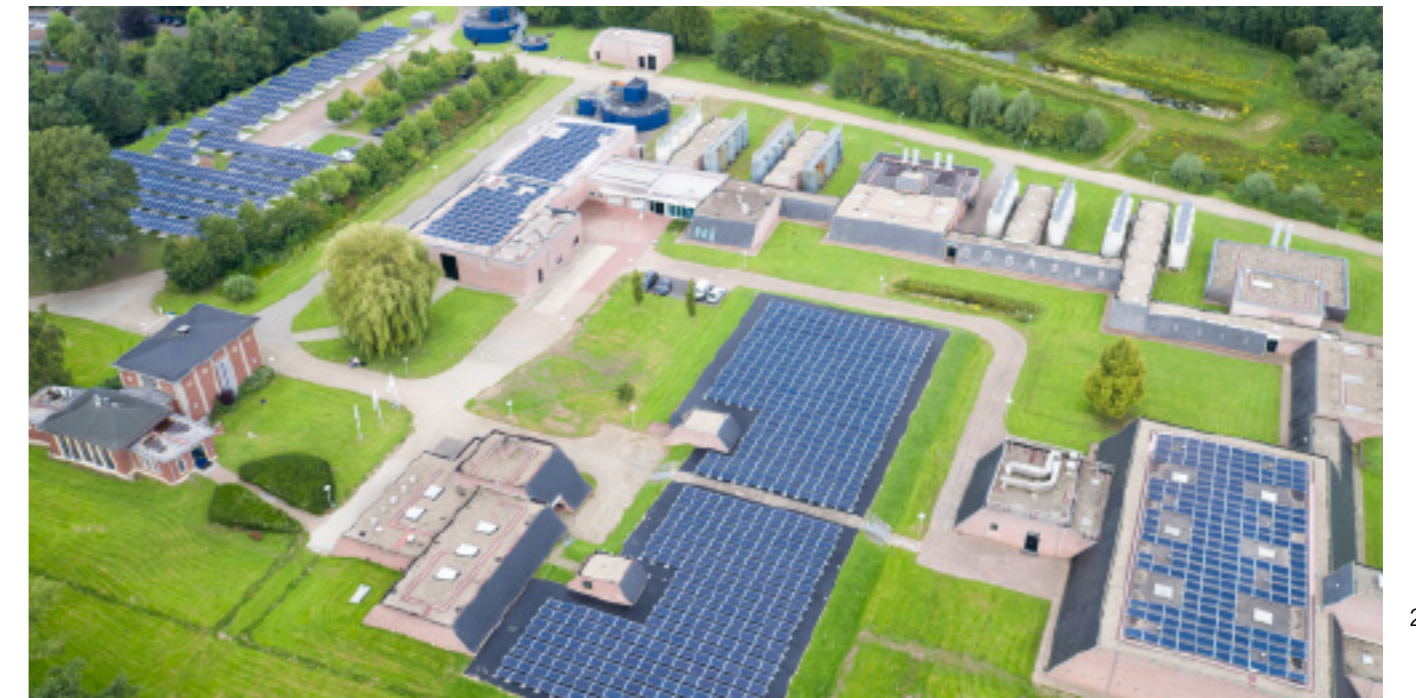
Vitens generates approximately 1.2 megawatts peak through 4462 solar panels at five sites. Shown below is the Engelse Werk production site.
