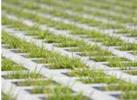
incidentele uitrit in grasbeton
